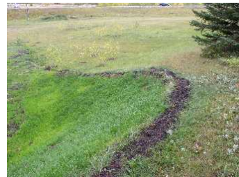
Blanket Installation and Result
